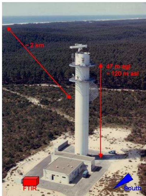
figure II.2.1-b : The HF Tower and surroundings.
